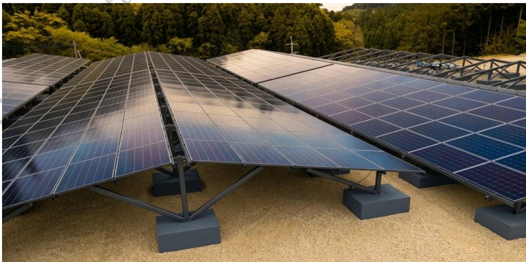
Figure 2.2: Isolated Concrete Footing
